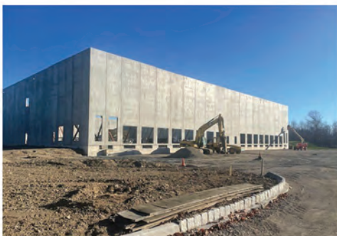
81 LEONARDS DRIVE TOWN OF MONTGOMERY, NY 80,000 Square Feet The Frassetto Companies
